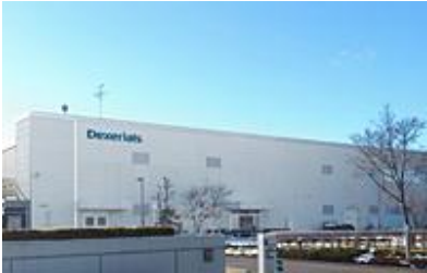
■ Dexerials Photonics Solutions Corporation Tome Operation (Miyagi)
